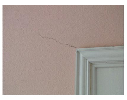
Figure 10 Drywall Crack
