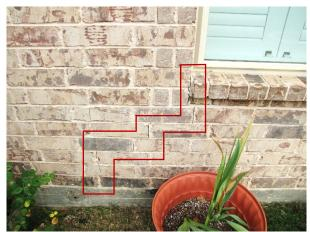
Figure 12 Stairstep Crack in Brick Veneer
