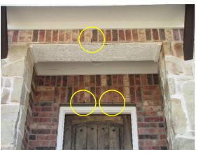
Figure 13 Weep Holes in Brick Veneer
